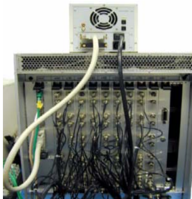
98 Channel ACP with TPD Caddy Installed
